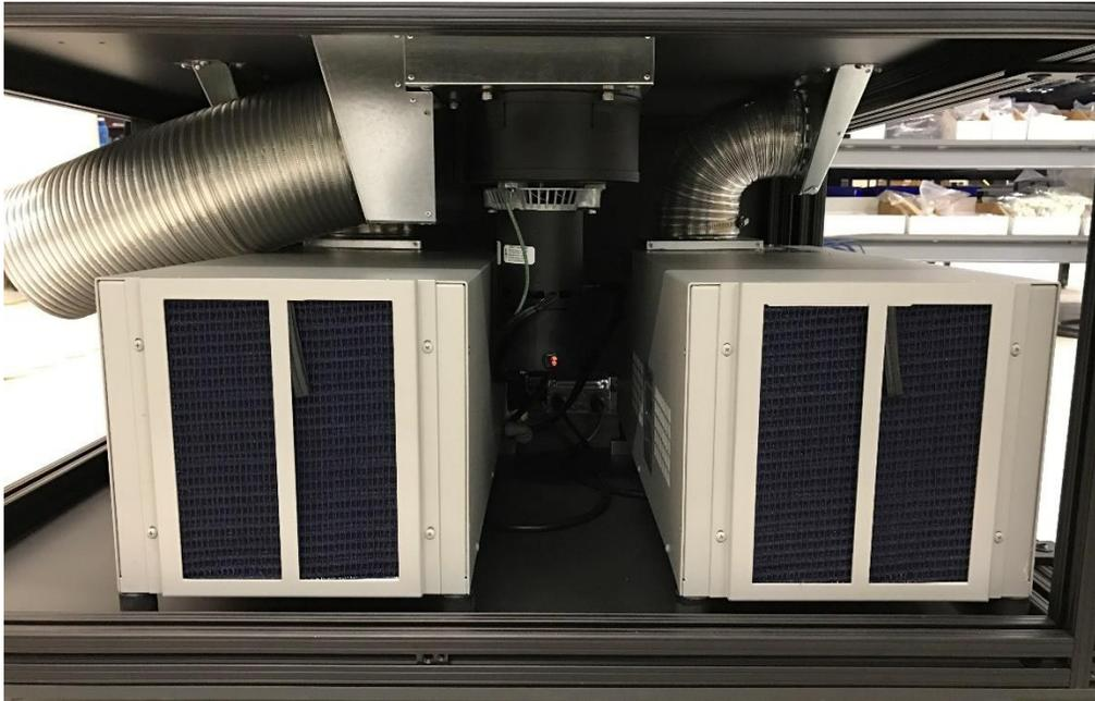
Figure B.1 Blower A/C Units under oven
