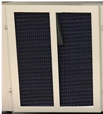
**Figure B.4** A/C Unit Air Filter
