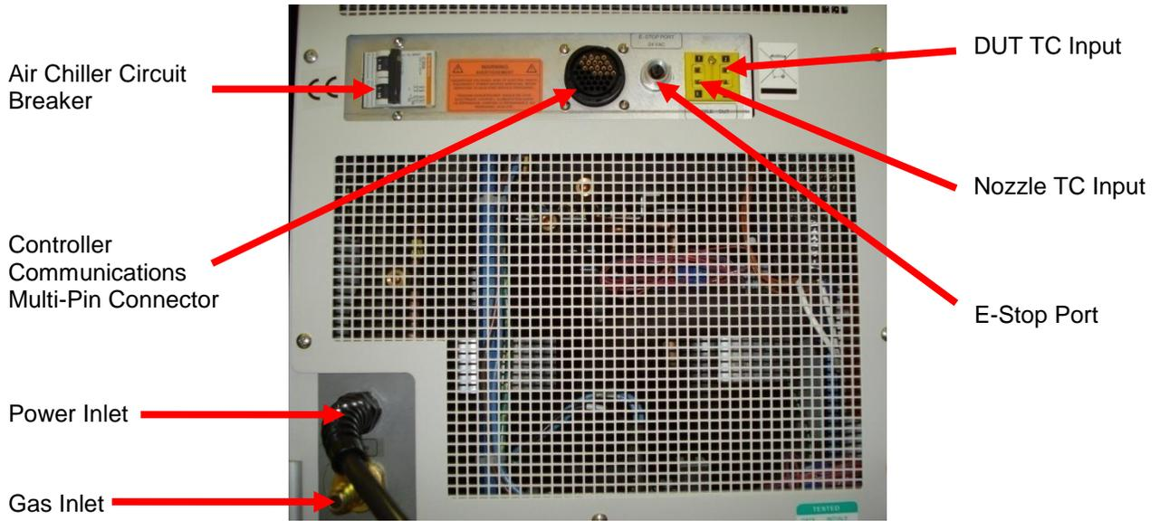
**Figure 1.5** Air Chiller Back Panel Connections
